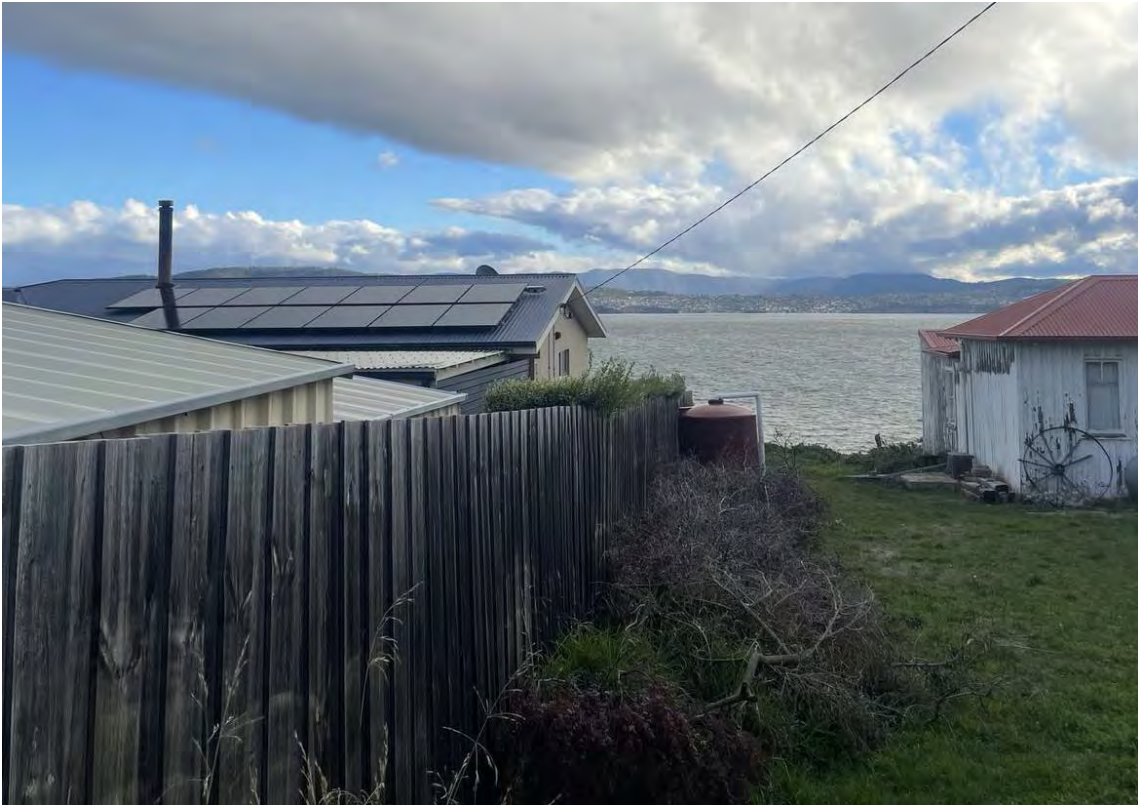
Image One: Shared boundary between 21 and 23 Gellibrand Lane, western elevation.
