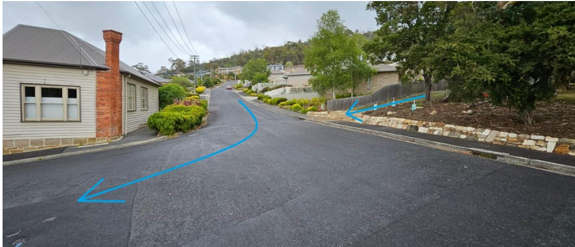
Figure 5: Diversion of Overland Flow at (Wellington - Moirunna Road) Intersection
