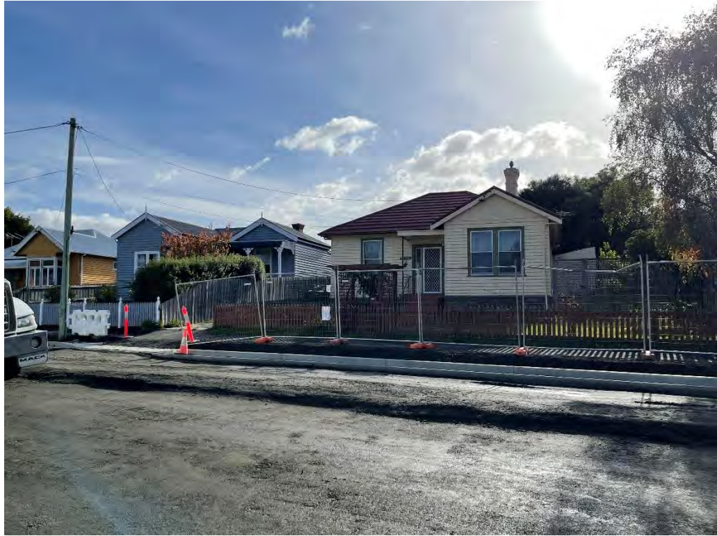
Figure 4. Existing frontage of 16 Douglas Street.
