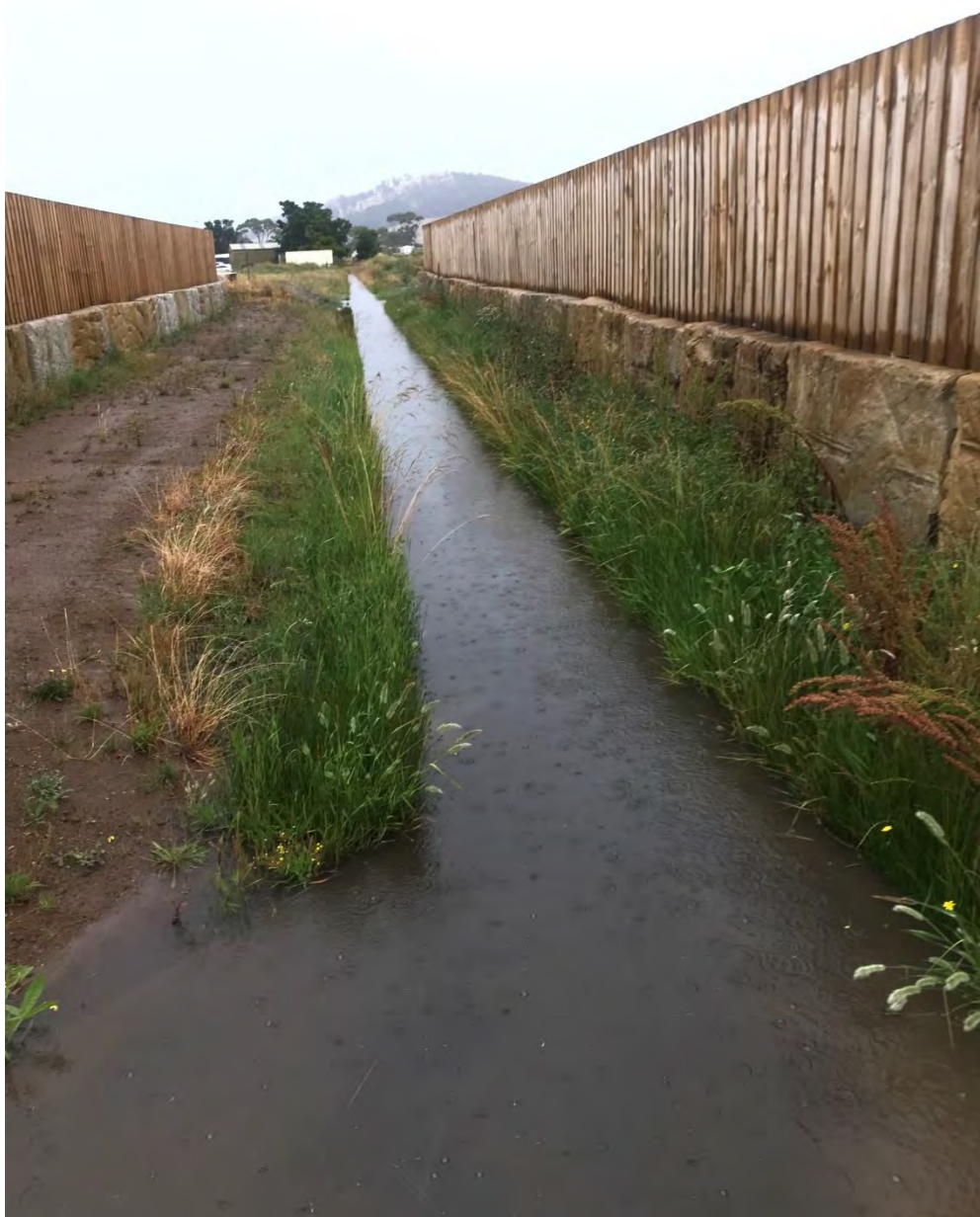
Photo 2 Drainage Channel and walking track on the southern side of Mannata Street. Photo take after a high rainfall event
