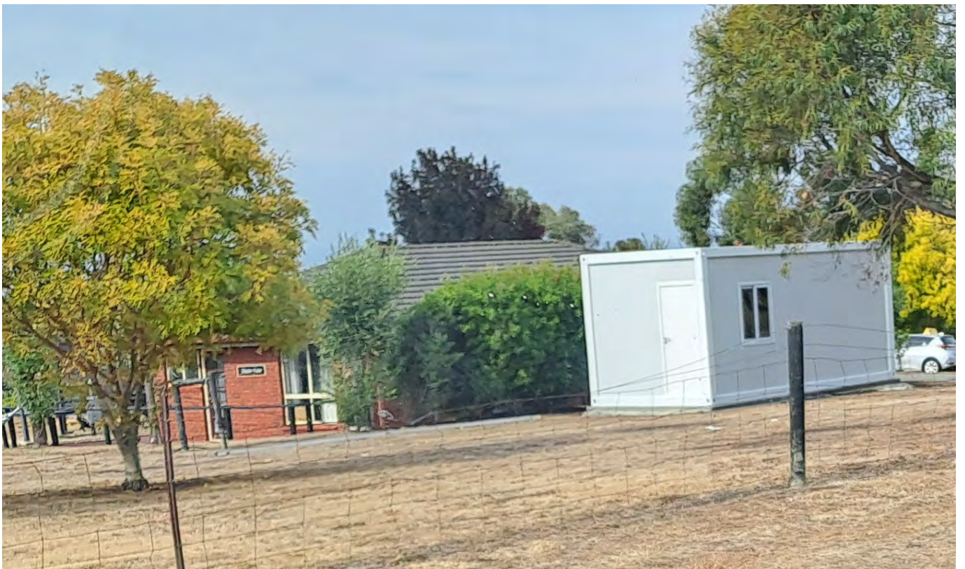
Image 2: view from Kelson Place of unapproved structure, looking north-east
