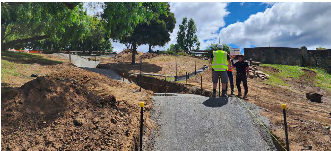
■ Works underway at the Richmond Riverbank Parklands.
