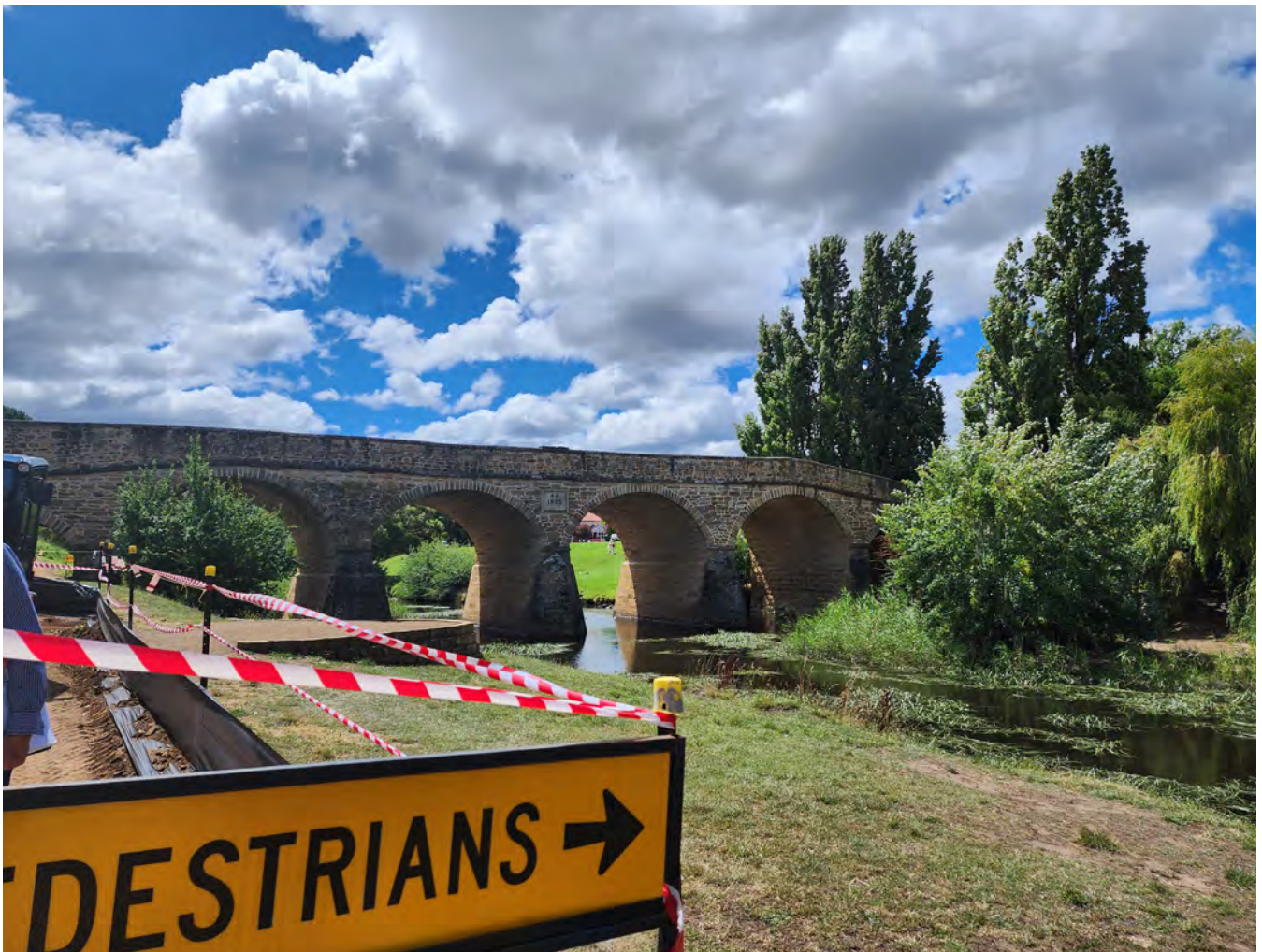
■ Works underway at Richmond Riverbank Parklands.
